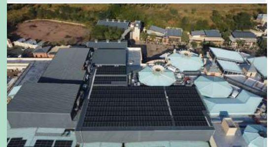
↑ Roof mounted panels
